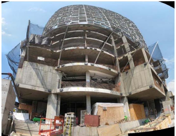
Figure 12: Photo showing portion of cantilevered balcony system
